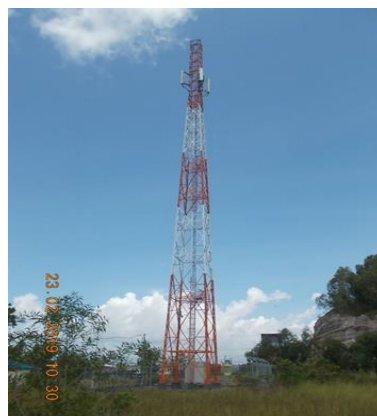
Figure 1. Self-Supporting Tower Source: Data in research, 2019
