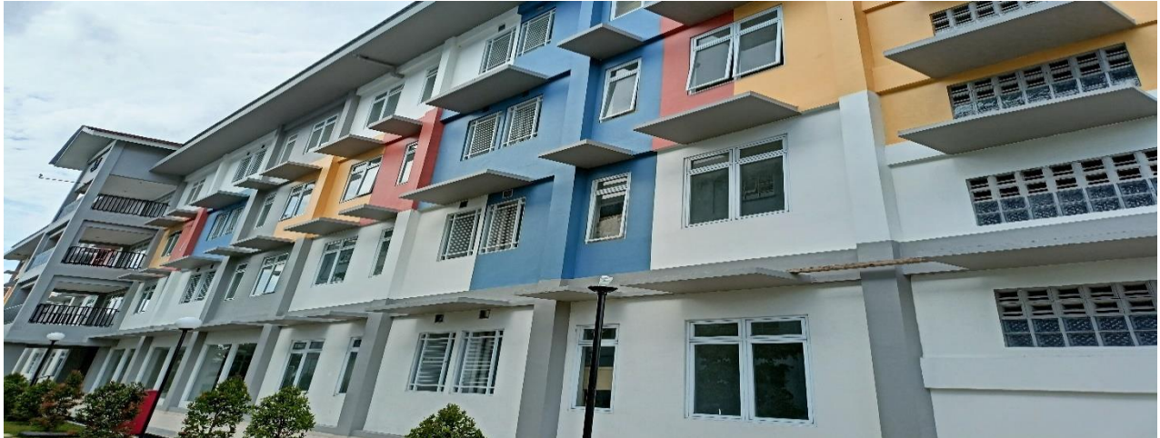
Figure 1. Workforce and Construction Work of Flats in Surabaya
