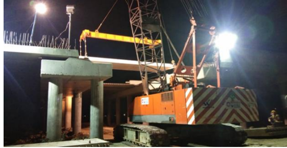
Figure 1. Tools Crawler Crane
